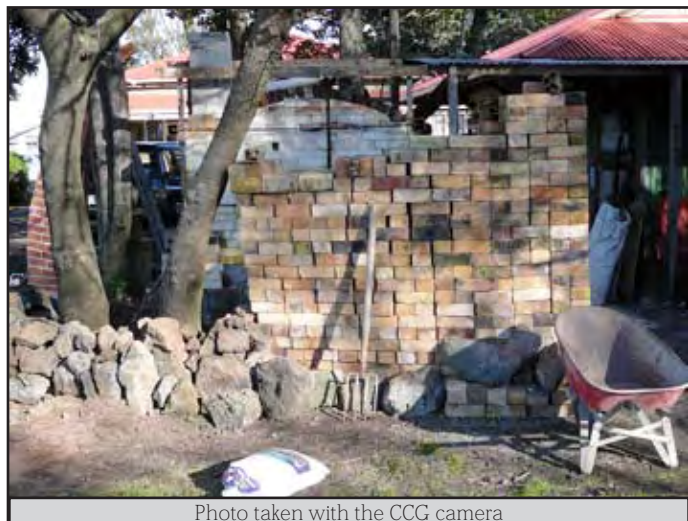
Photo taken with the CCG camera
